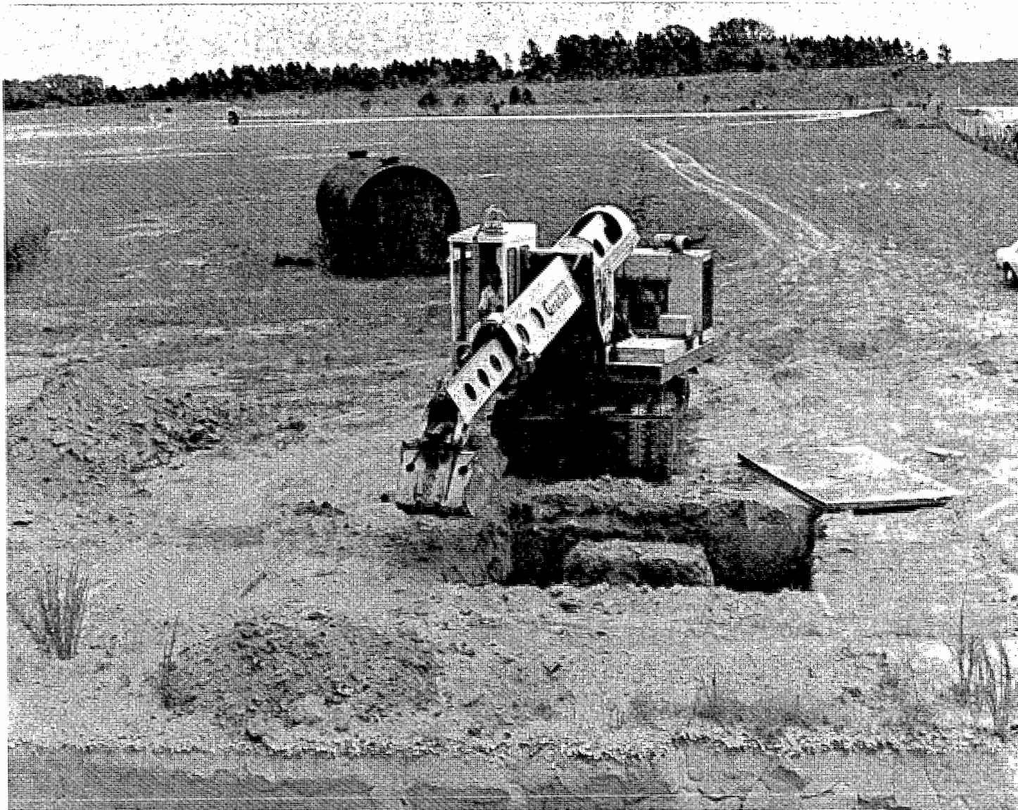
FIGURE 14. Excavation of Lysimeter Pit
