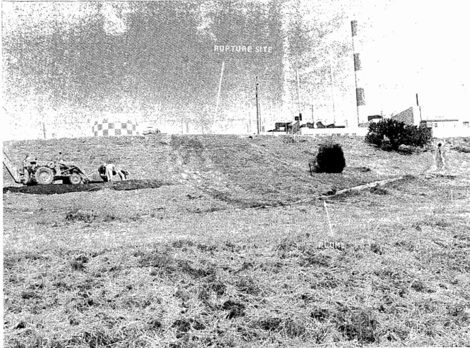
FIGURE 36. Hillside Below Pipeline Rupture Site Near the Waste Disposal Building
