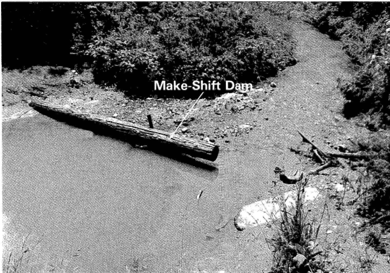
FIGURE 10. South Canal Viewed from the Top of the Earthen Dam
