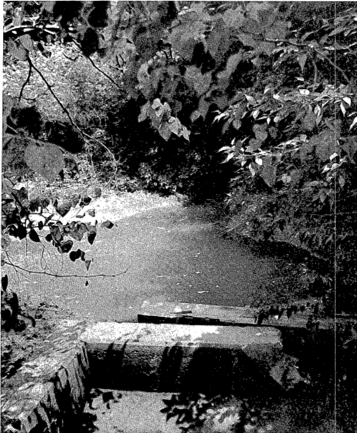
FIGURE 16. - Water in the South Canal as it enters the overflow creek as viewed from the Cincinnati Dayton Road.
